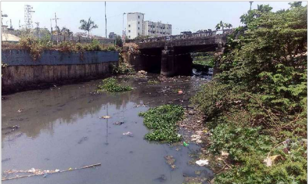
VIEW TOWARDS UPSTREAM
